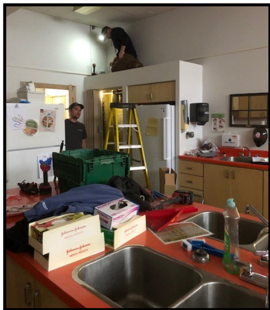
New wiring in Kitchen
